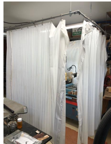
The curtains are hung from the ceiling using 1/4" all-thread rod and 3/4" Electrical metal Tubing (EMT)
